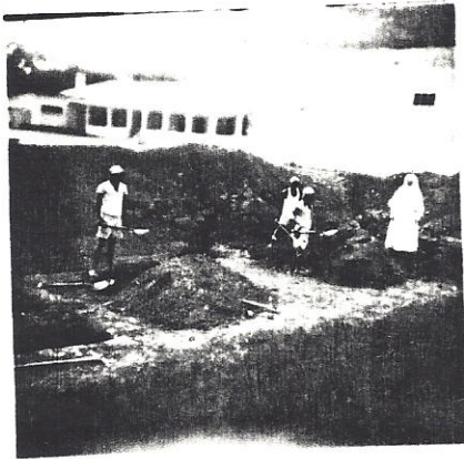
Work on the second hostel begins. (Block I)
